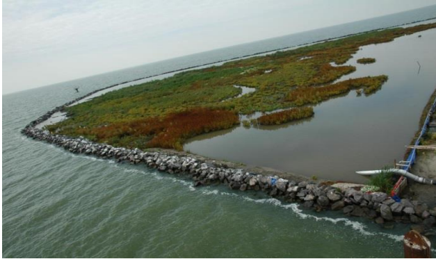
Constructed wetlands, use excessive sediments
